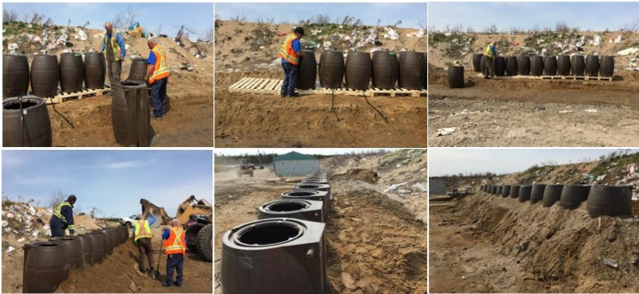
*Picture 1. Photographs showing preparation of berm and setting up rain barrels for experimentation*
